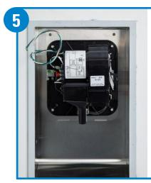
Knock out the appropriate electrical inlet on dryer wall plate and install dryer insides onto dryer mounting plate using all 6 mounting nuts supplied.
