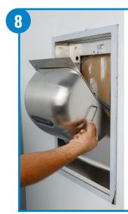
Install dryer cover with 2 flat head tamper proof bolts using special wrench provided.
