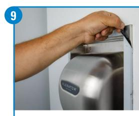
Return dryer to upright position and refasten to Wall Box using the 2 button head tamper proof bolts. Remove protective film from Wall Box. Turn on power and test for proper operation.
