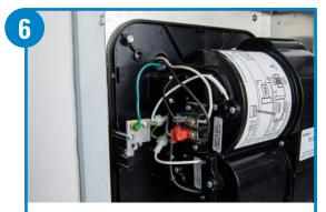
Connect electrical service to Terminal Block of hand dryer. Properly ground the dryer via the supplied ground screw.
