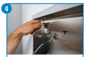
Re-fasten dryer mounting plate to Wall Box using the 2 button head tamper proof bolts previously removed.
